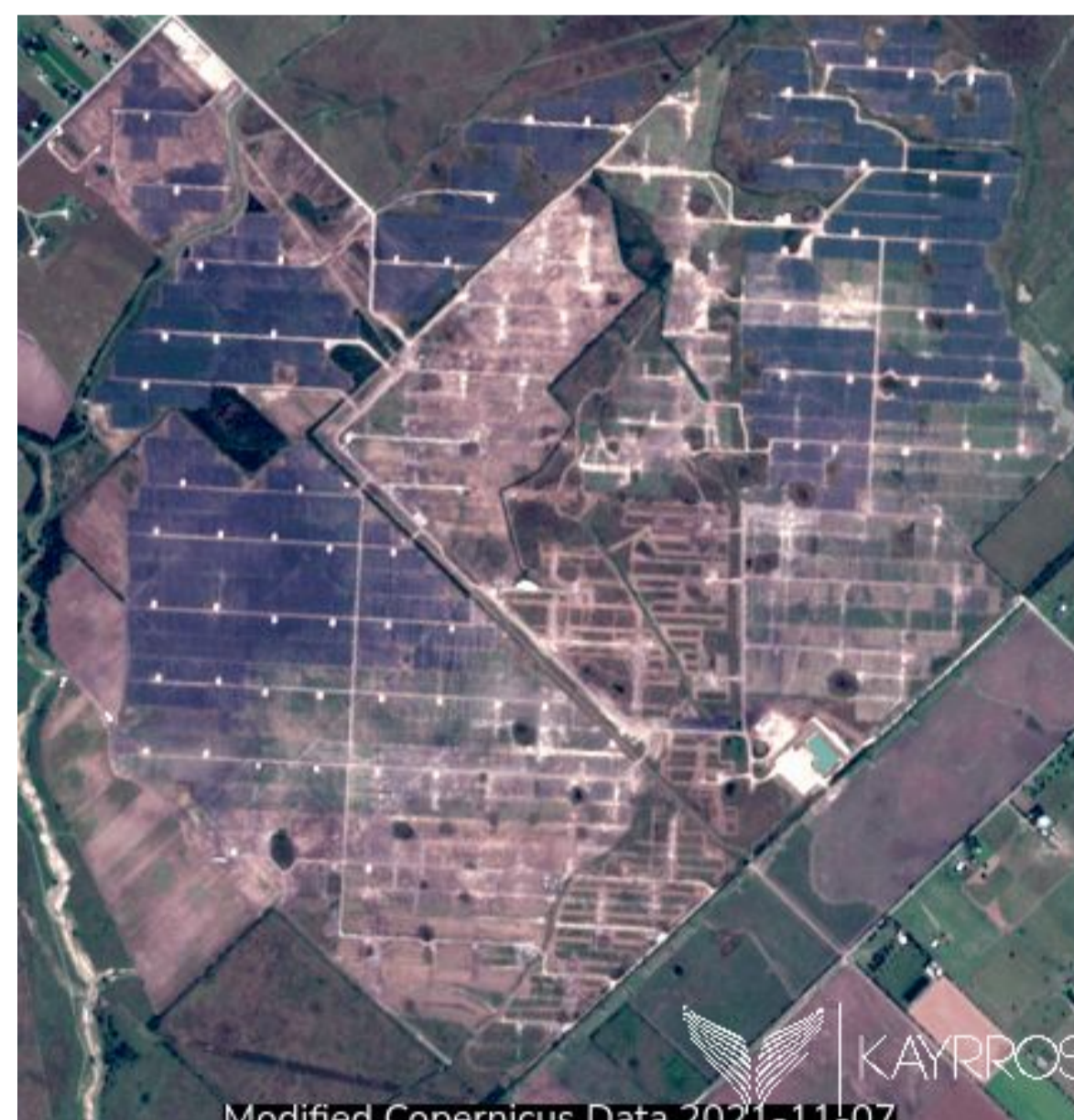
Solar Project completions
